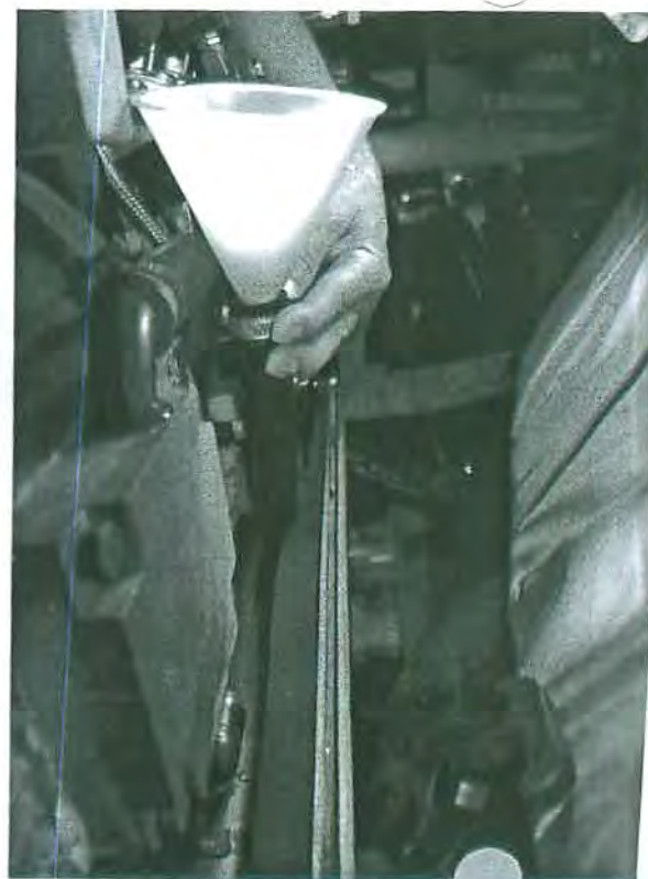
Heat exchanger tube configured to accept rydlyme marine. Note the large tube attach point just below the rectangular zinc and above the heat exchanger itself.
