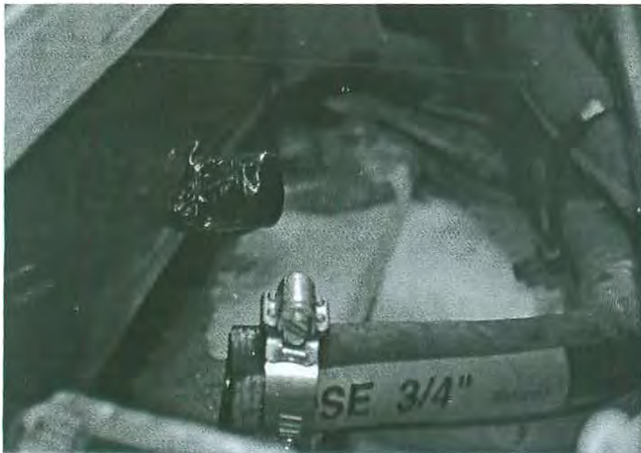
Raw water inlet tube removed & taped closed
