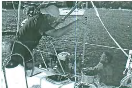
Installation of temporary straps for vertical support.
