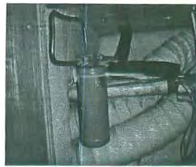
RFD and piping behind locker
